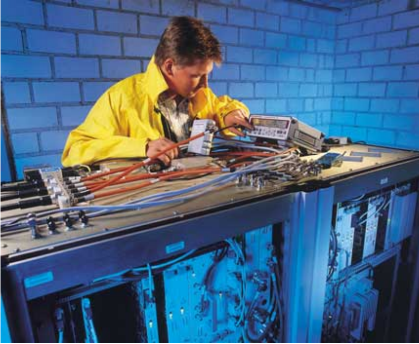
NRT during installation of a mobile radio base station
